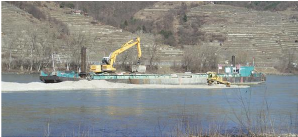
Figure 8: Artificial island building at the Danube River
